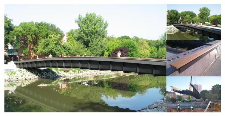
The Almuñecar footbridge is built with innovative materials that minimize the weight and height of the structure. The structure consists of a single carbon fiber U-girder fixed at the abutments, with a height of 1.20 m, a width of 4.0 m and an approximate length of 40.0 m.
